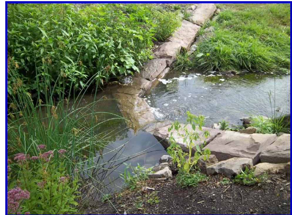
One of two rock cross veins directs flow to the center of the stream to protect the bridge structures.
